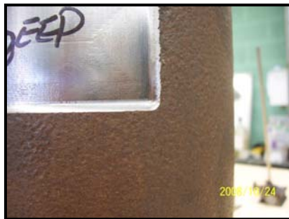
b) Photograph of corrosion patch
