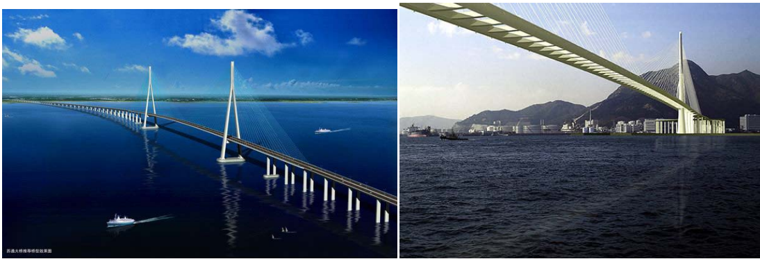
Figure 1-1 Sutong Bridge (Left) and Stonecutter Bridge (Right)
