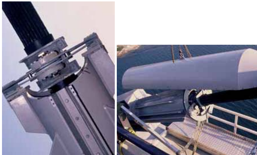
Figure 2-11 Friction damper installed on Uddevalla bridge in Sweden
