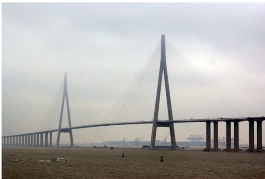
Figure 4-1 Sutong bridge –Jiangsu Province ,China
