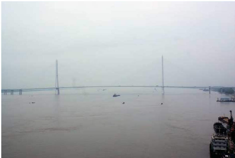
Figure 4-8 Third Nanjing Yangtze Bridge
