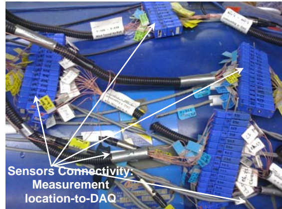
w. Instrumentation and System Insulation-2
