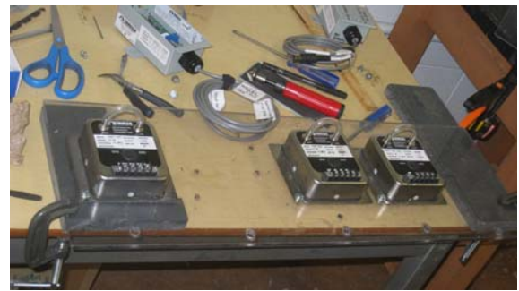
p. Airside Pressure Transducers Wiring
