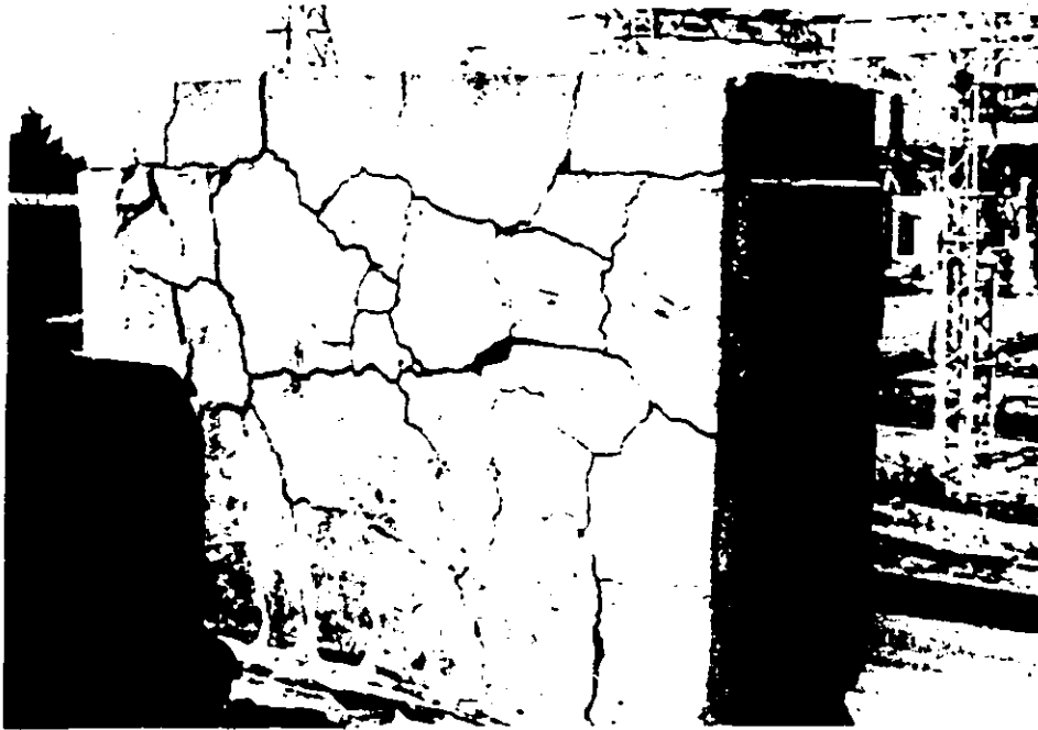
Figure 2.3: Portion of the Beahurnois Dam, Quebec, constructed with reactive alkali-silica aggregate (Potsdam sandstone) showing pattern and map cracking. (Photo by Dr. Peter Hudec, 1986).
