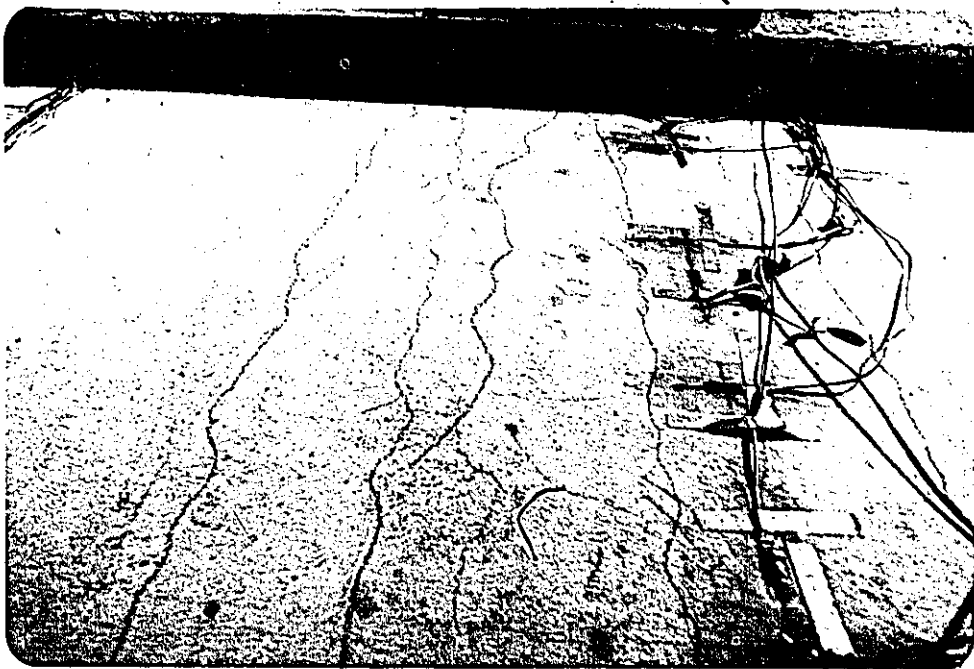
FIGURE 6.19 TRANSVERSE CRACKS AT THE INTERMEDIATE SUPPORT ON THE LEFT SIDE OF LOADED BEAM, BRIDGE MODEL (I), (AT LOAD OF 50 KIPS).
