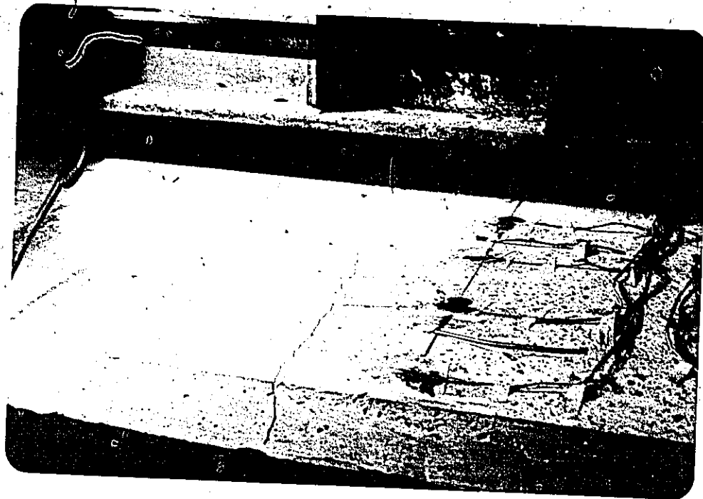
FIGURE 6.21 TRANSVERSE CRACK AT THE INTERMEDIATE SUPPORT, BRIDGE MODEL (II), AT LOAD OF (180KIPS).
