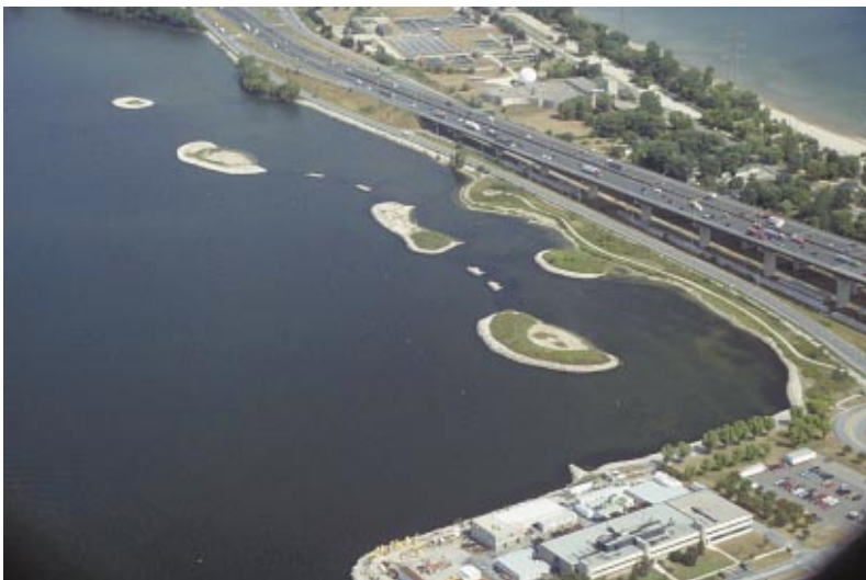
Figure 29 The Northeastern shoreline of Hamilton Harbour following island construction and enhancement of the shoreline using soft engineering techniques. Note the traditional shoreline at the top.
