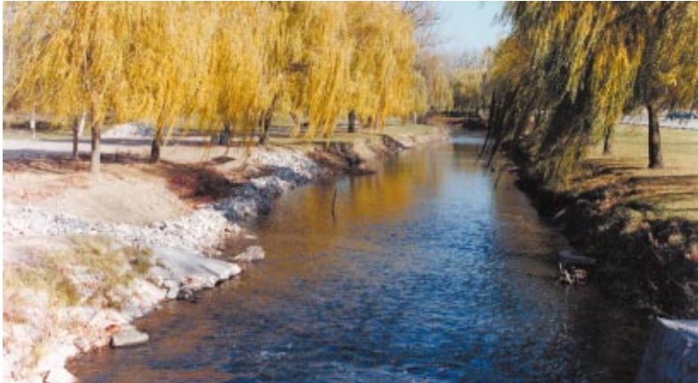
Figure 36 The soil bioengineering workshop construction area on the north (left) side of the Rouge River. Existing unstable streambank conditions are illustrated on the south (right) side.
