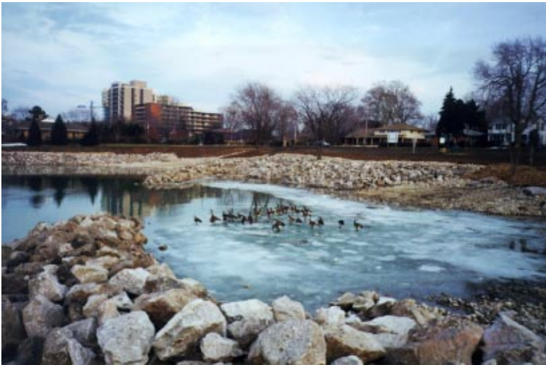
Figure 22 Goose Bay Park enhancements, such as rock groynes, were undertaken to improve fish spawning and refuge habitat.
