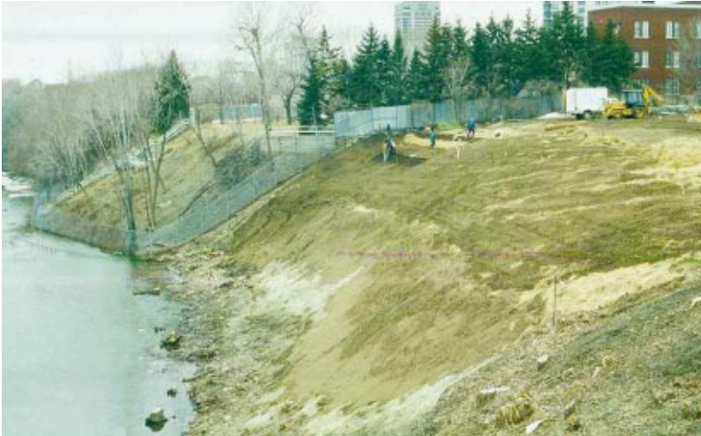
Figure 11 Placement of live fascines on contour with erosion control fabric along the Jacques Cartier Park.
