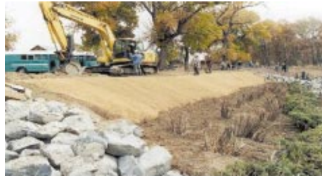
Figure 33 Willow clumps with Juniper Tree Revetment at the toe.
