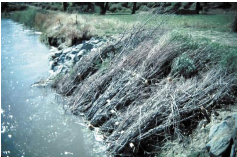
Figure 32 Installation of a brush mattress to reduce accelerated erosion.
