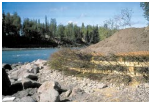
Figure 14 Overhanging cover was provided by live siltation and live cribwall constructions along the Kenai River.
