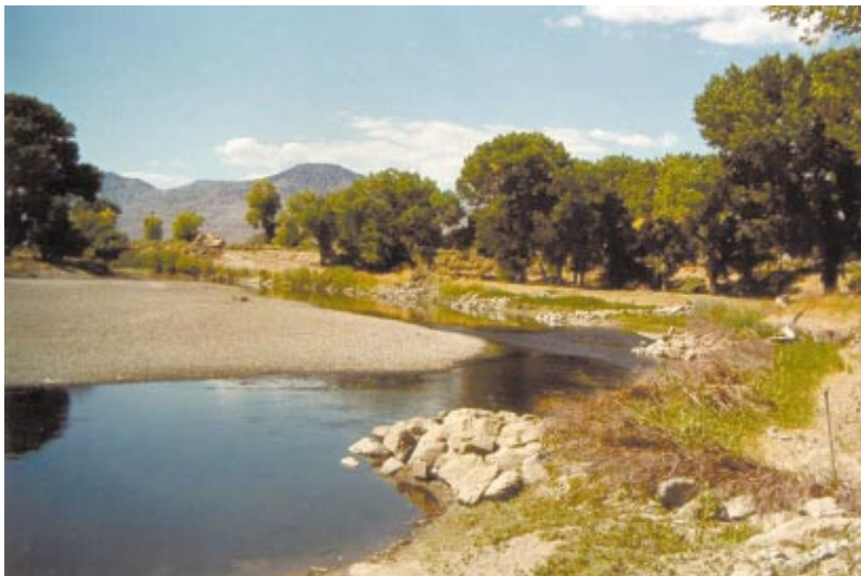
Figure 35 A view of the project site looking upstream about 10 months after construction.
