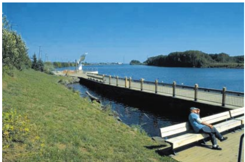
Figure 44 The open pile construction of this scenic overlook provides instream cover for aquatic habitat and increased public access without destroying or degrading the existing wetland areas along the shoreline.
