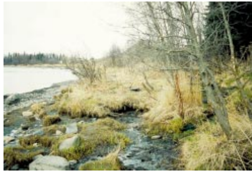
Figure 13 Rapid streambank erosion caused by heavy public use along the Kenai River in Alaska.
