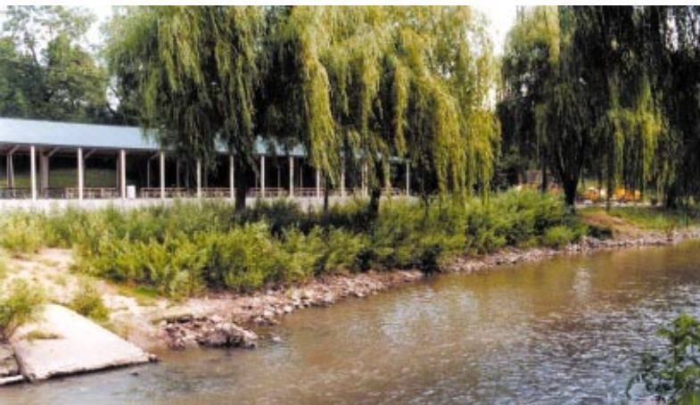
Figure 38 The workshop construction area where the three various techniques were used after one season of growth.
