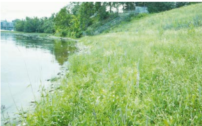
Figure 12 Vegetated shoreline resulting from the use of bioengineering techniques in Jacques Cartier Park.
