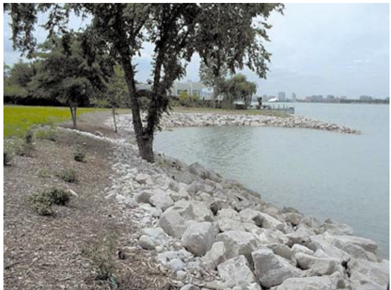
Figure 21 Goose Bay Park shoreline, after rehabilitation, is protected from erosion and enhanced for fish and wildlife habitat.
