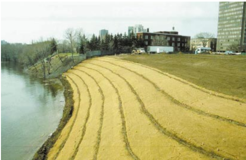
Figure 11 Placement of live fascines on contour with erosion control fabric along the Jacques Cartier Park.
