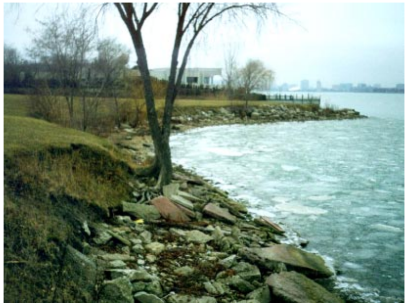
Figure 20 Goose Bay Park shoreline, prior to rehabilitation, was badly eroding.
