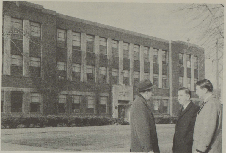
Discussing plans for the renovation of Memorial Hall to a closed circuit television classroom building are, from the left: William Morgan, director of engineering services at the University; Walter Romanow, director of communication services; Esio Marozotto, technician.
