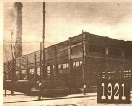
THE FORMER POWER HOUSE as it looked in 1921. We are still using this building. Now the engine and material testing laboratories, payroll, printing and the industrial relations division are housed there.
