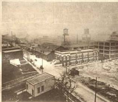
SIX-STOREY BUILDING under construction. Note the river, which has been chased back a bit since.
