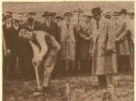
W. R. Campbell breaks ground for the new Foundry in 1934.
