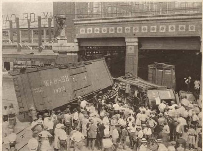
LESS SERIOUS THAN IT LOOKS was this collision between a street car and a freight car outside the crane-way of Plant 1 on August 17, 1922. No one was seriously hurt, although several street
