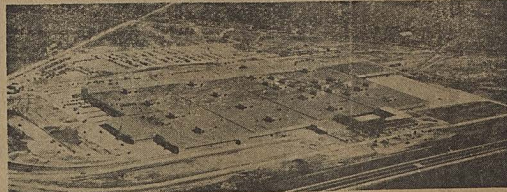
THE FIRST CAR has been turned out by this new Ford of Canada 224-acre assembly plant at Oakville, Ont. The largest industrial building under one roof in Canada, the plant moved into production only one year after the first steel girder was erected. The new building places Ford of Canada assembly operations in the heart of the Canadian market.
