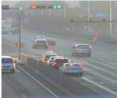
Figure 2-7. TSCT installed at traffic signals in China. (Source: Yu and Shi, 2015)
