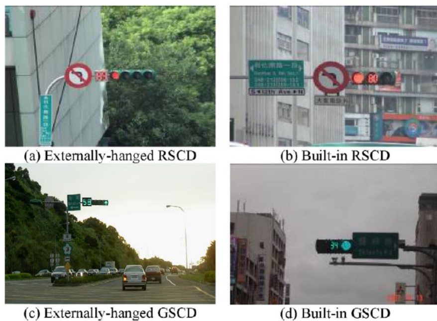
Figure 2-3. TSCT installed at traffic signals in Taiwan. (Source: Chiou and Chang., 2010)
