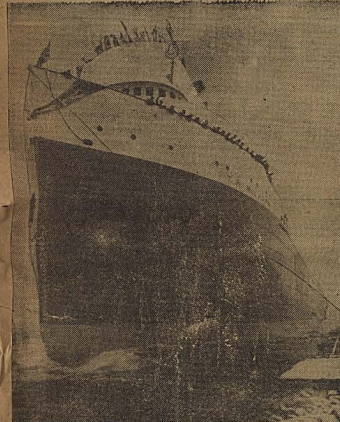
The T. R. McLagan, named after the president of Canada Steamship Lines, slides down the ways at Midland, Ont., into the waters of the Georgian Bay. The 716-foot inland waterways freighter is the largest ship of her type in the world and was the biggest shipbuilding event in Midland's history.
