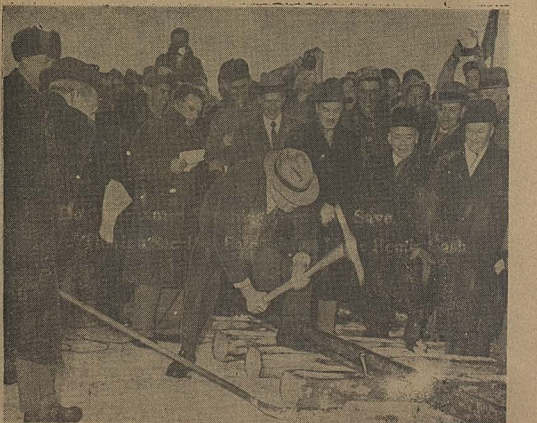
Donald Gordon, chairman and president, Canadian National Railways, drives the last spike at Lynn Lake, Manitoba, to officially open the new 144-mile line from Sheridon northward.
