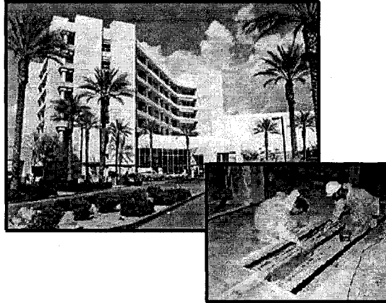
Fig. 2-13: St. Joseph's Hospital, Arizona (Strengthening of the floors with CFRP plates)
