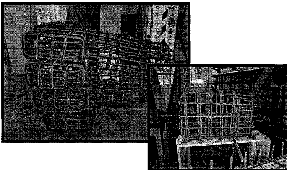
Fig. 3-16: Preparation of reinforcement
