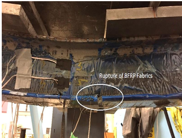
Figure 2.14: Failure mode showing rupture of BFRP
