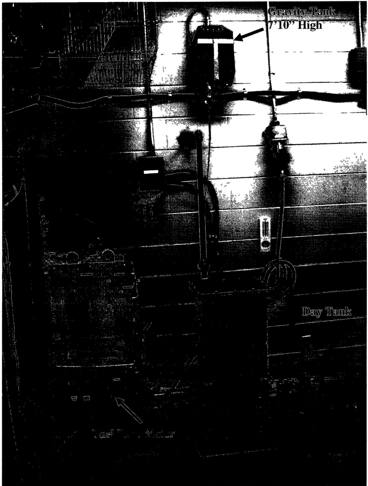
**Figure 3.13 Gravity Tank Setup**
