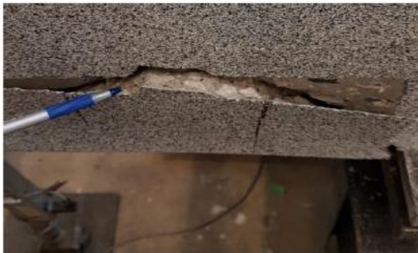
Figure 5.18: Shear-tension failure of strengthened beam (Hughes, 2018)
