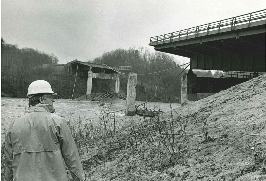
Figure 1.1: Schoharie Creek Bridge collapse in NY, 1987 (Croyle 2017)
