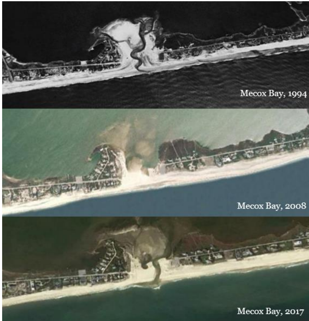
Figure 9: Annual breaching at Mecox Bay, Long Island, New York, to prevent property flooding.
